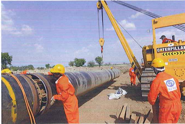
Figure 2. Line pipe fit-up for mainline welding.
