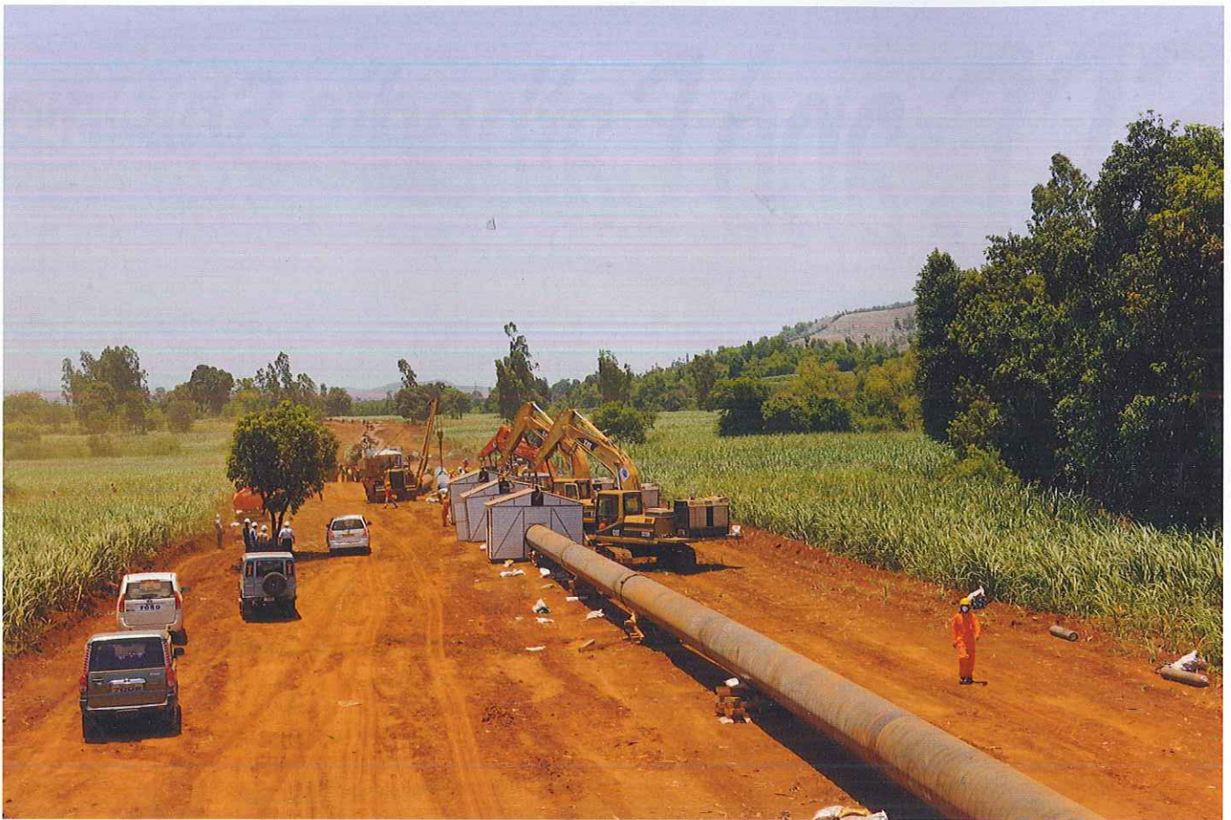
Figure 3. Automatic welding in progress.
