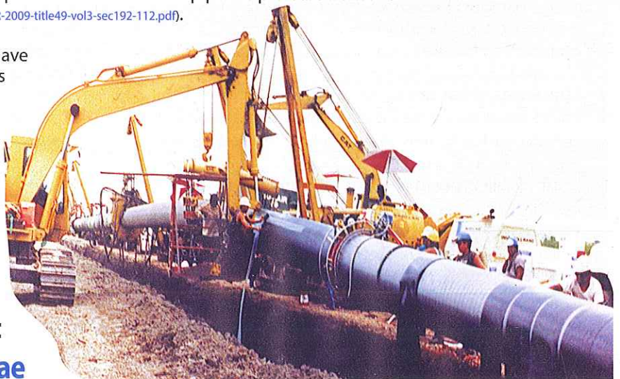
1990 - A 36" natural gas line rehabilitation using RD-6.
